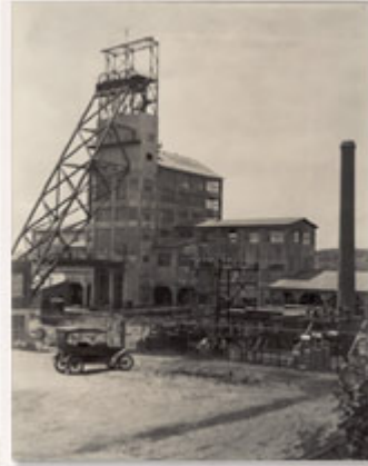
In 1923, the Fuller shaft of the Retsof Salt Mine was nearing completion.
