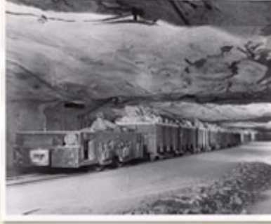
A miner removed salt by electric rail car in the mid-1930's. In the earliest days, mules pulled the carts of salt out of the mine.
