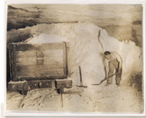
At the turn of the century, miners used shovels to fill carts with rock salt. All bagging was done by hand as well.
